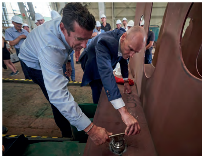
▲ The commencement of the construction of the RV Anna Weber-van Bosse at Armon Shipyards in Vigo on 11 October 2023, was marked with the symbolic welding of the ‘coin for good luck’ by Gert-Jan Reichart and Henk Oenema on behalf of NIOZ. (Image courtesy: NIOZ)
