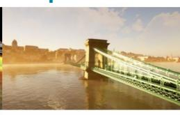
Two Hungarian companies designed a three-step data collection workflow to overcome the challenges in this urban surveying project in Hungary, which included the use of UAVs and remotecontrolled boats for Lidar and photogrammetry data. The result: a digital 3D BIM-compatible model of Budapest's iconic bridge over the River Danube to assist in preparations for restoration and renovation work.
