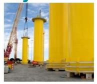
DONG Energy, leading partner in the construction and operational phases of the Walney project, uses Holmatro's aluminium hydraulic cylinders for levelling the foundations of the turbines. So-called transition pieces (TP's) are mounted on top of monopiles driven into the seabed, together forming the foundations.
